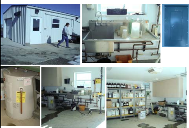
Bldg #8417 – Chemical Storage/Handling Facility
