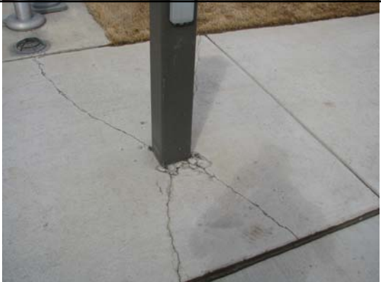
Cracking Concrete (Poured 2013) around new building #8415.
