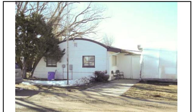
Bldg #8404 – Laboratory (Two Attached Greenhouses and their footprints are in the process of removal. They were recently sold. On)
