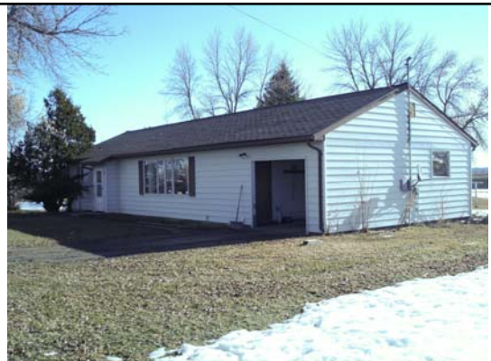
Bldg #8403 – Foreman Residence
