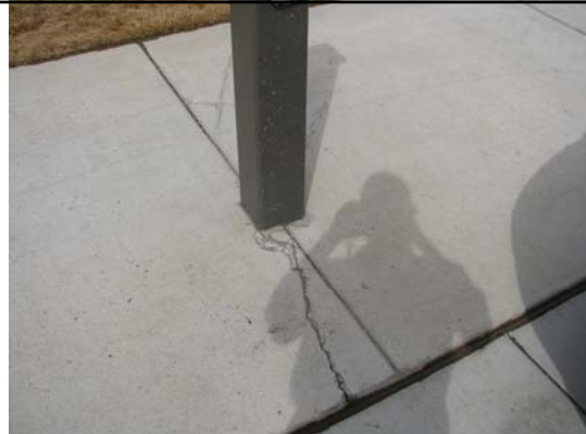
Cracking Concrete (Poured 2013) around new building #8415.
