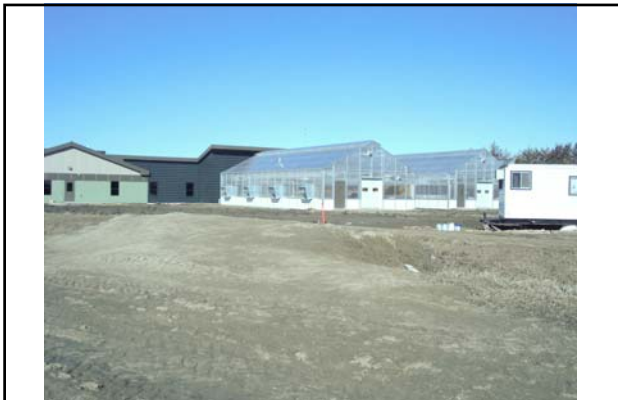
Bldg #8415 – Main Offices with Lab Classrooms, Meeting Room, Labs, 2 Greenhouses (East side)
