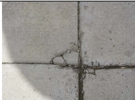
Cracking Concrete (Poured 2013) around new building #8415.
