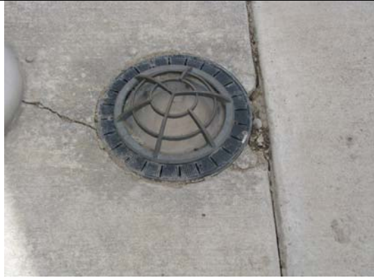
Cracking Concrete around new building #8415
