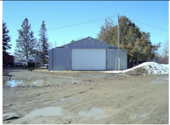
Bldg #8410 – Machinery Shed
