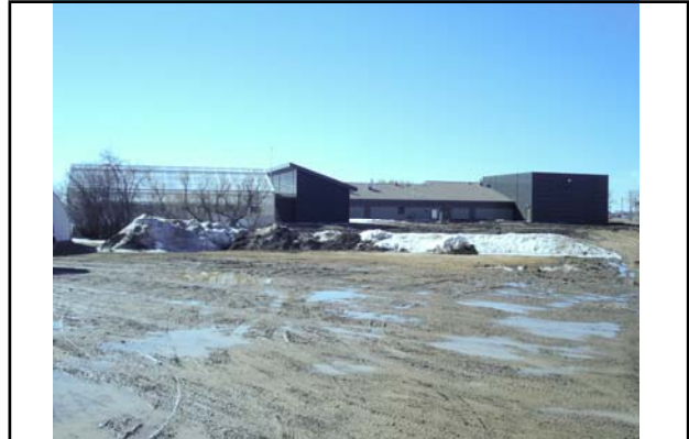
Bldg #8415 – Main Offices with Lab Classrooms, Meeting Room, Labs, 2 Greenhouses (North side)
