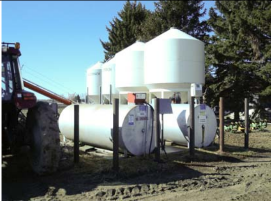
Bldg #8414 – Seed Bins; Bldg #8418 - Fuel Tanks
