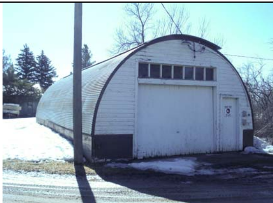
Bldg #8402 – Cold Storage (Old Chem Storage – likely to be demoed)
