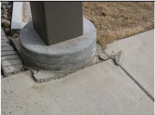
Cracking Concrete (Poured 2013) around new building #8415.
