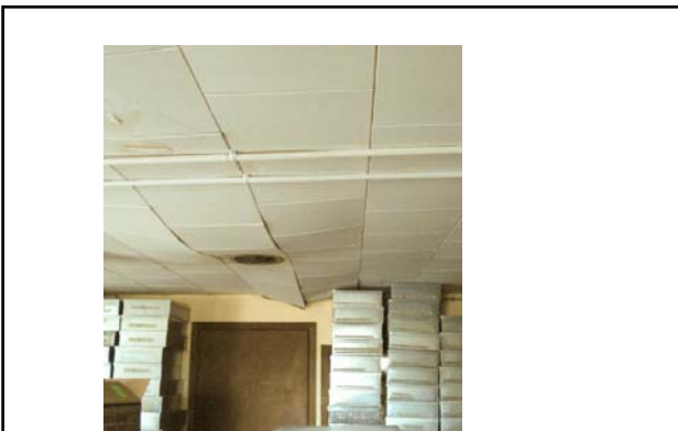
Bldg #8404 – Laboratory (attached to Bldg #8411 – Two Greenhouses)
