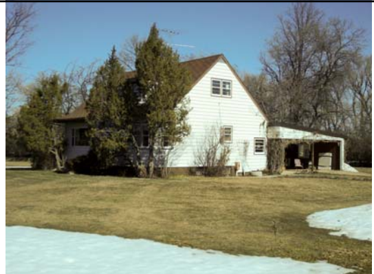
Bldg #8401 – Superintendent Residence
