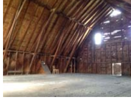
Bldg #802 – Lutz Farm Cow Barn
