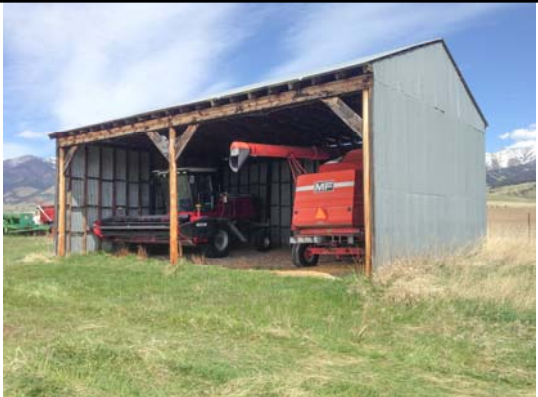
Bldg #811 –Machine Shed
