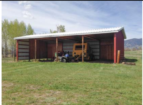
Bldg #812 –Machine Shed
