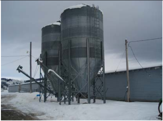
Bldg #741 – Grain Bins
