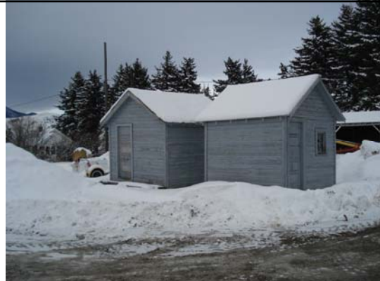
Bldg #731 Store House (on left) and Bldg #740 Oil House (on right)
