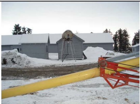
Bldg #731 Store House (on right) and Bldg #740 Oil House (on left)
