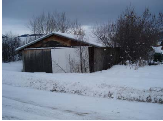
Bldg #754 – NE Wooden Shed #2
