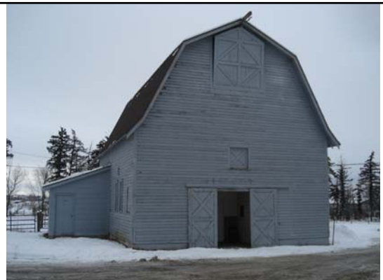
Bldg #722 – Horse Barn / Lab
