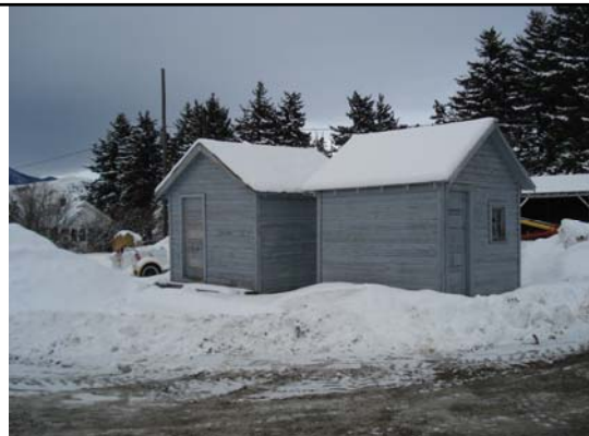
Bldg #740 Oil House (on right) and Bldg #731 Store House (on left)
