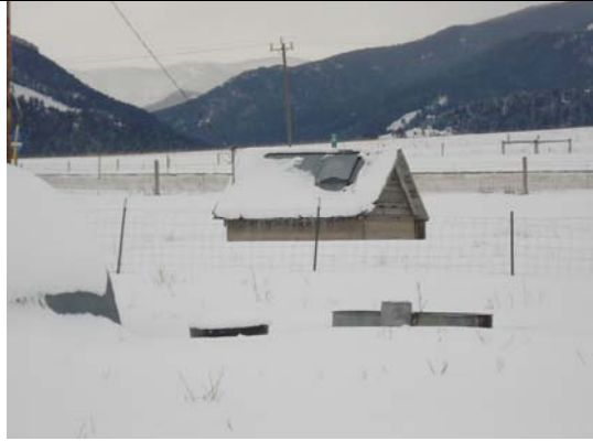
Bldg #743 – Pump House
