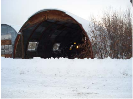
Bldg #753 – NE Quonset Shed #2
