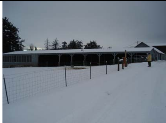
Bldg #737 – Ram Test Shed
