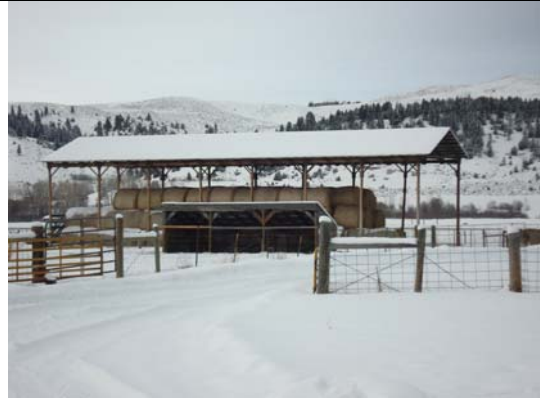
Bldg #735 – Hay Shelter (in back) and Bldg #733 – Sheep Shelter (in front)
