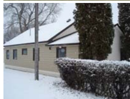
Bldg #7406 – Horticulture & Soils Lab
