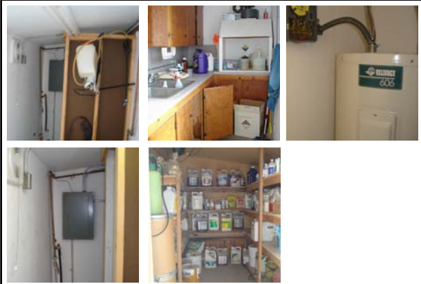
Bldg #7411 – Pesticide Shed / Handling Facility
