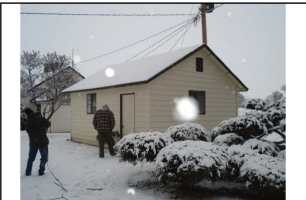
Bldg #7415 - Bio Control Handling Facility
