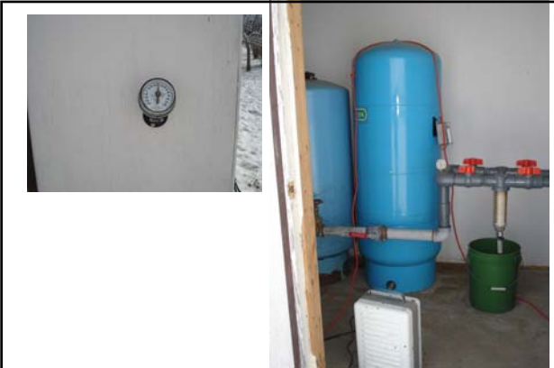
Bldg #7412 – Pump House
