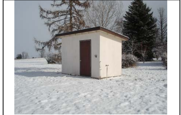
Bldg #7412 – Pump House
