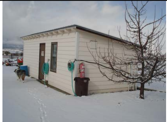
Bldg #7411 – Pesticide Shed / Handling Facility
