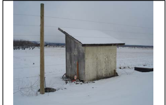
Bldg #7413 – Pump House #2
