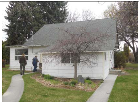
Bldg #7401 – Bio Laboratory/Lunch Room
