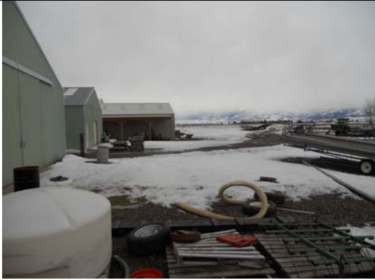
Eastside shot of buildings – bldg #s 727, 704, 703
