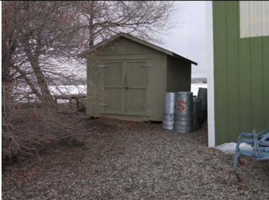
Shed – No bldg #
