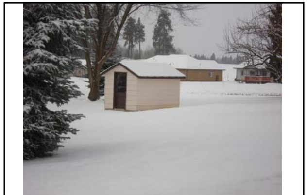
Bldg #6413 - Miscellaneous Storage
