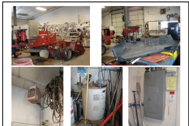
Main shop of Bldg #6411 - Shop
