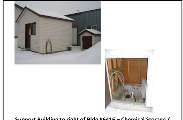
Support Building to right of Bldg #6416 – Chemical Storage / Handling Facility
