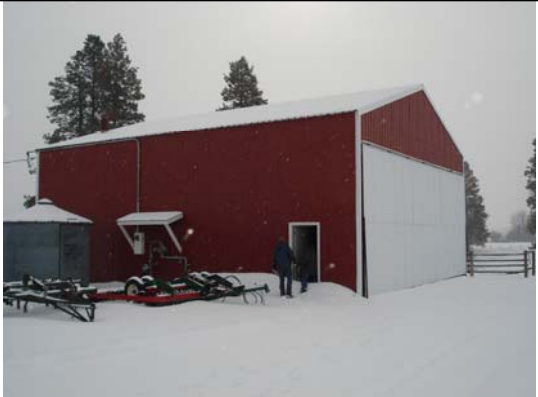
Bldg #6412 - Research Distillation Facility
