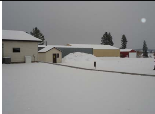
looking south East toward Bldg #s 6408, 6416, 6410, 6417, 6412
