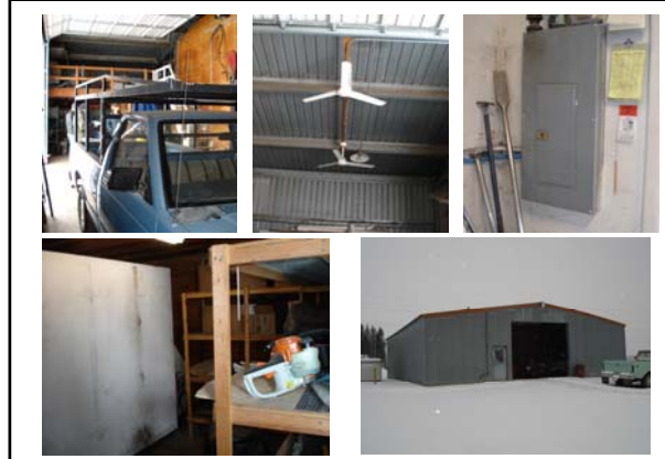
Unheated part of Bldg #6411 - Shop
