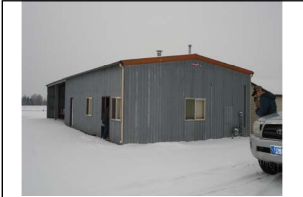
Bldg #6410 – Garage / Two Wet Labs
