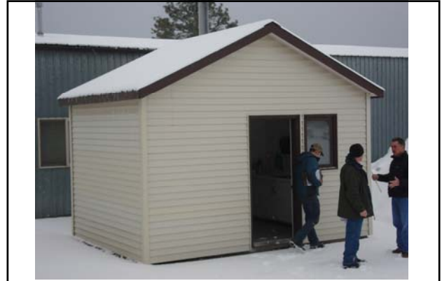
Bldg #6416 – Chemical Storage / Handling Facility
