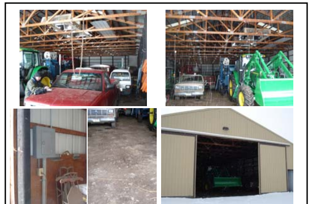
Bldg #6417 – Machine Shed
