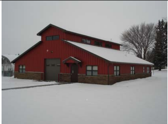
Bldg #6426 – Seed & Plant Processing Research, Wet Lab
