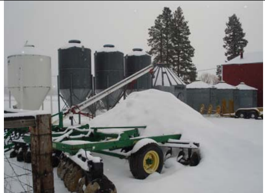
Grain Silos left to right: Bldg #s 6427, 6407 (three bins), 6423, 6428 (three bins)
