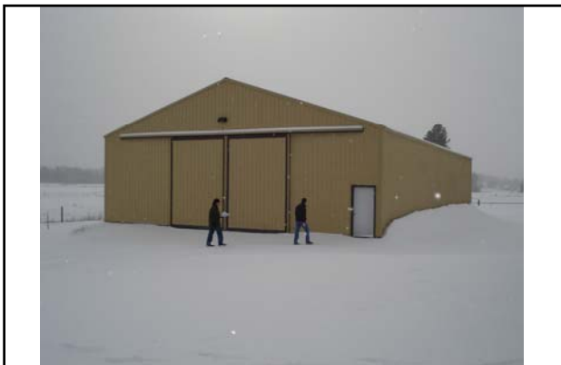
Bldg #6417 – Machine Shed
