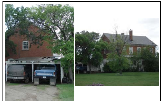
Bldg #5401 – Living Quarters Apt 9
