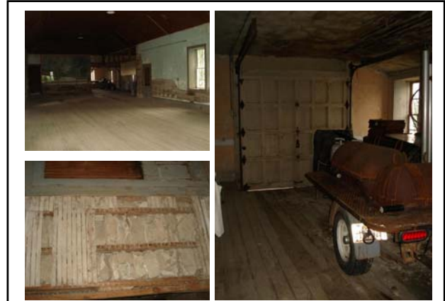
Bldg #5409 – Garage #1 (Amusement Hall)
