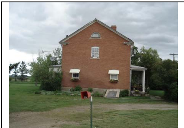
Bldg #5401 – Living Quarters Apt 9
