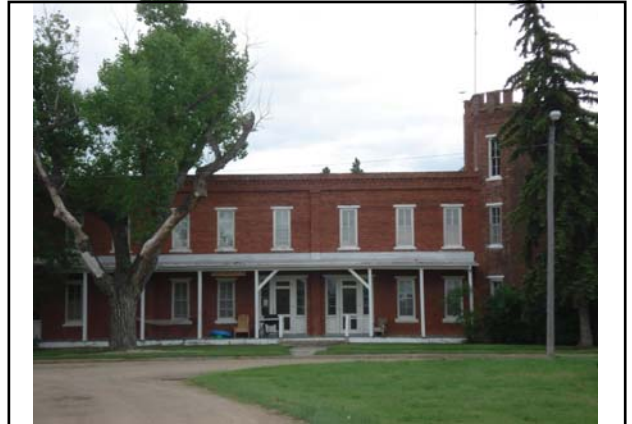
Bldg #5403 – Six Unit Apartment
