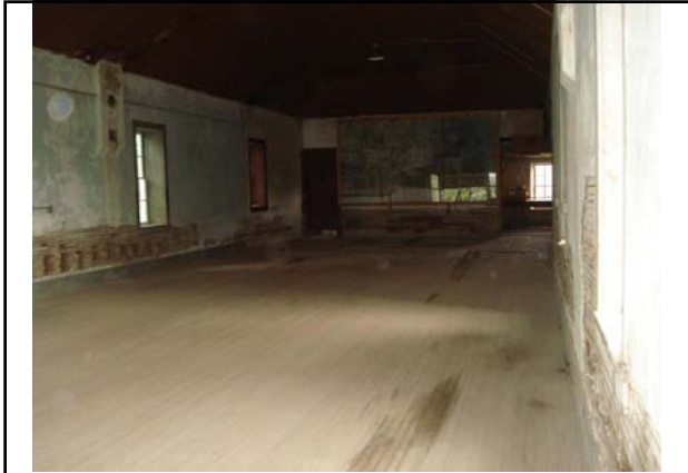
Bldg #5409 – Garage #1 (Amusement Hall)
