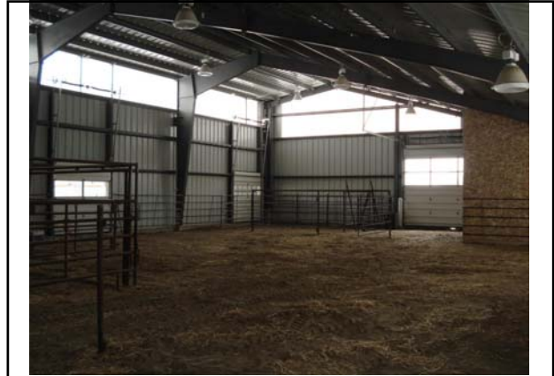
Bldg #5467 – Upper Calving Barn
