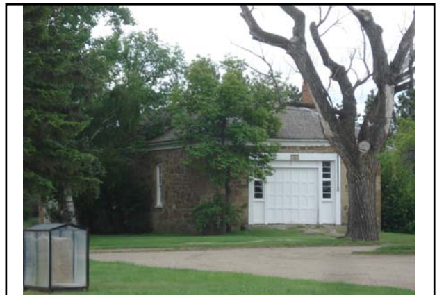
Bldg #5409 – Garage #1 (Amusement Hall)
