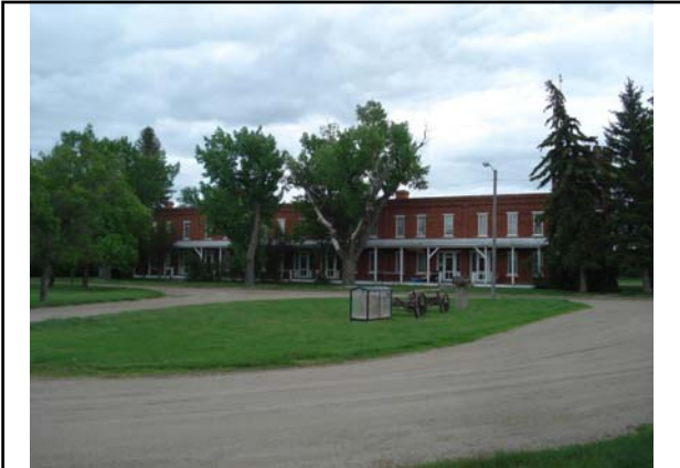
Bldg #5403 – Six Unit Apartment
