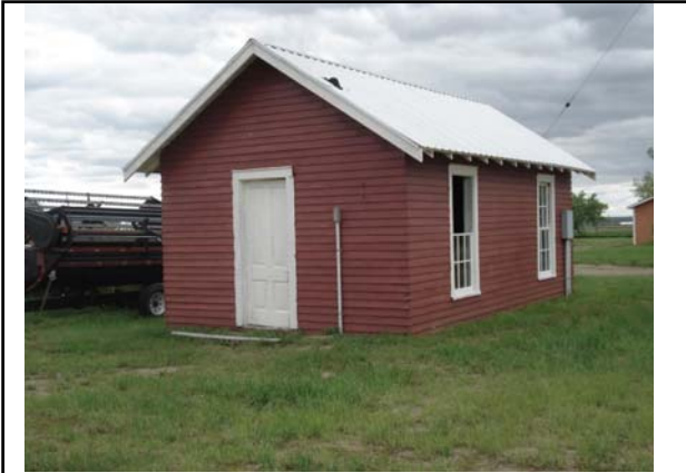
Bldg #5413 – Pump House
