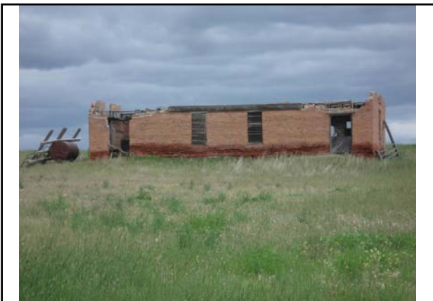
Bldg #5416 - Hog House – Inactive and Not Maintained
