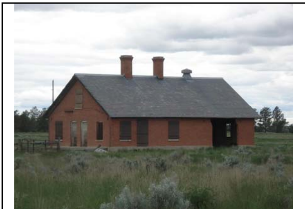
Bldg #5420 – West Guard House (maintained by hist society)
