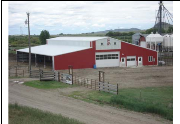
Bldg #5467 – Upper Calving Barn
