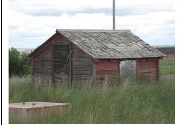
Bldg #5424 – Valve House
