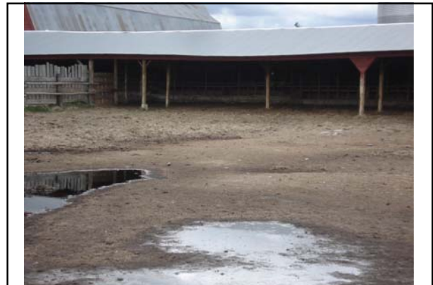
Bldg #5410 – Research Steer Barn
