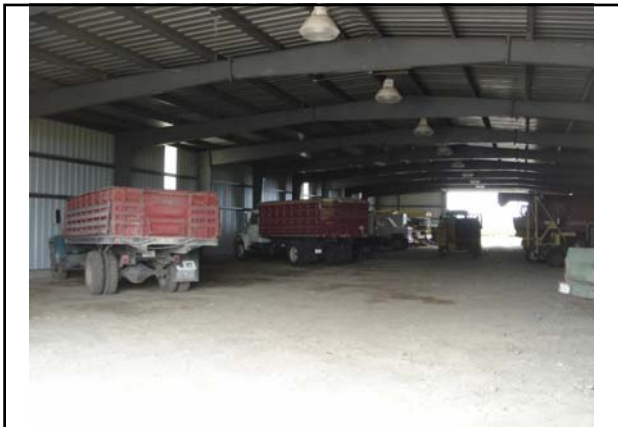
Bldg #5426 – Machine Storage Shed
