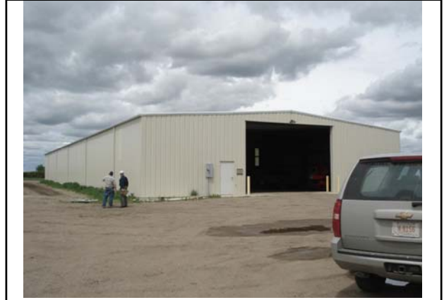
Bldg #5426 – Machine Storage Shed
