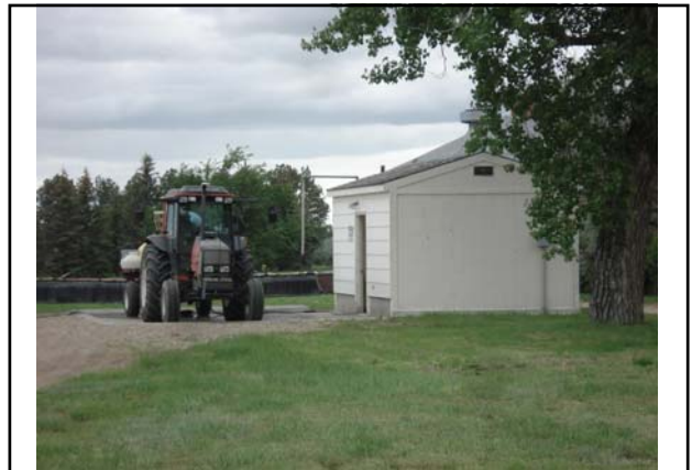
Bldg #5430 – Pesticide Storage/Handling Facility
