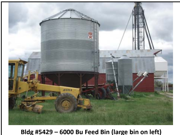
Bldg #5429 – 6000 Bu Feed Bin (large bin on left)
