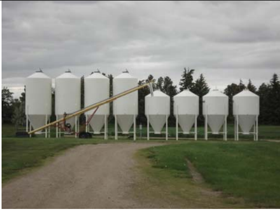
Bldg # 5436, 5437 – Four 250 Bu bins on right, Bldg #5438, 5439 – Four 400 Bu bins on left
