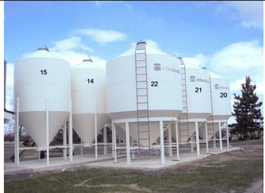
Part of Bldg #4431 – 3 of 5 Wheatland bins 20 to 22
