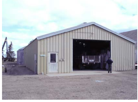
Bldg #4422 - Seed Processing Plant
