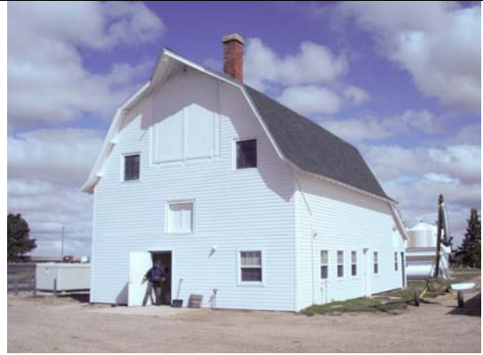
Bldg #4413 – Analytical Research Lab (was Dairy Barn)
