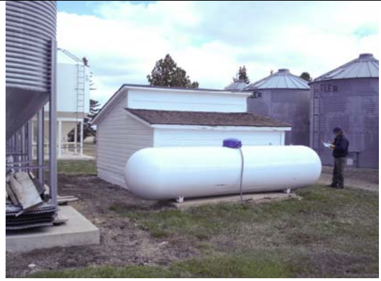
Bldg #4417 - Fertilizer Shed with Unnumbered Propane Tank
