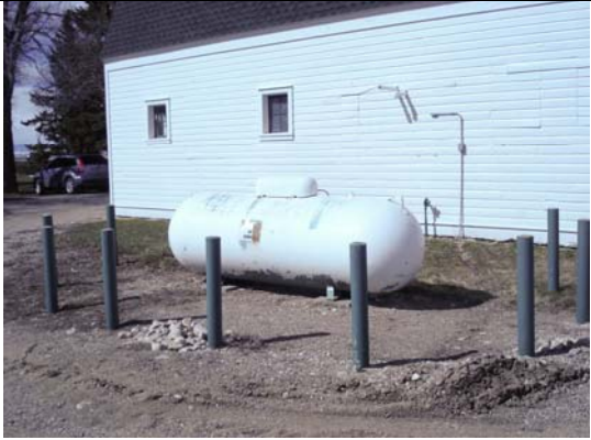
Propane Tank next to Bldg # 4409
