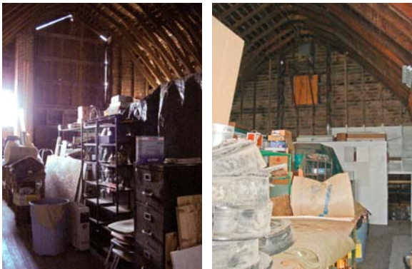
Bldg #4413 – Analytical Research Lab (was Dairy Barn)
