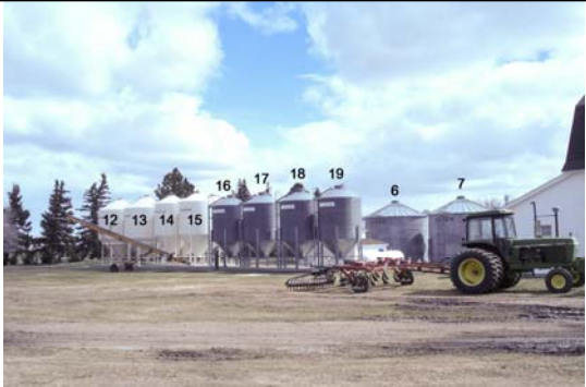
Part of Bldg #4431 – 2 of 5 Wheatland bins 12 to 13; Bldg #4430 –Wheatland bins 14 to 15; Bldg #4432 –Brock grain bins 16 to 19
