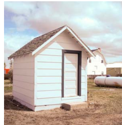
Bldg # 4405 – Well House
