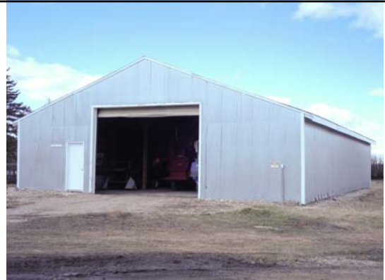
Bldg #4426 – Pole Machine Storage Shed
