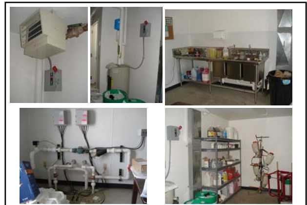
Bldg #4434 – Pesticide Handling / Shop
