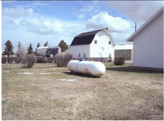
Bldg #4413 – Analytical Research Lab (was Dairy Barn)
