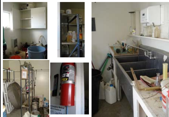
Bldg #4427 – Chemical Storage / Handling Facility
