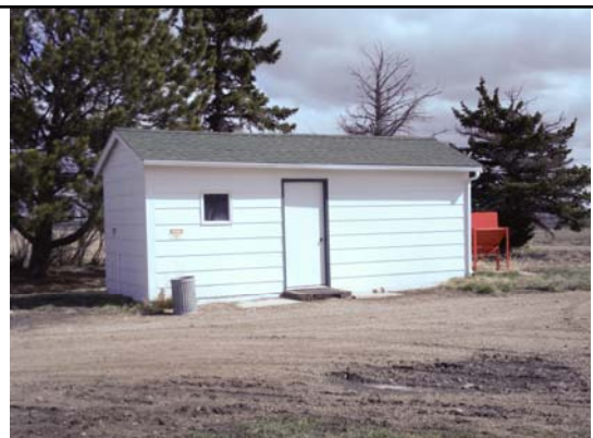
Bldg #4427 – Chemical Shed
