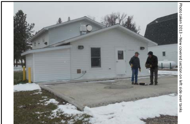
Bldg #4434 – Pesticide Handling / Shop
