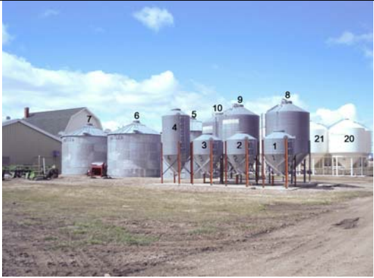
Bldg #4423 – bins numbered 1 to 4; Bldg #4424 – bins numbered 5 to 7
