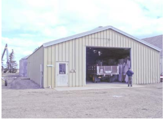
Bldg #4422 – Seed Processing Plant
