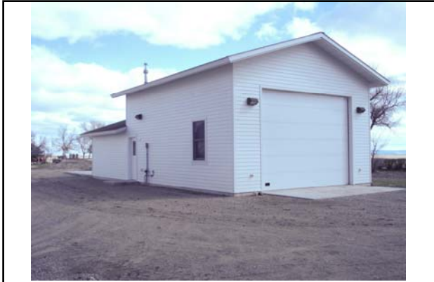
Bldg #4434 – Pesticide Handling / Shop
