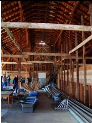
Bldg #3465 - Southern Annex Barn Complex
