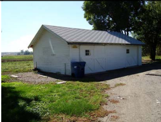
Bldg #3424 - West Residence Garage
