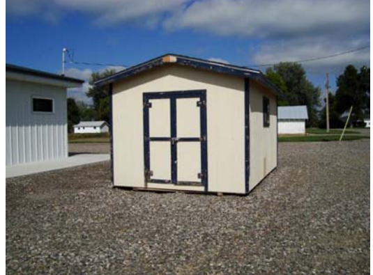
Bldg #3469 – Shed Next to Chem Wet Lab
