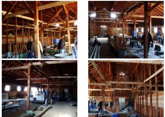
Bldg #3465 - Southern Annex Barn Complex
