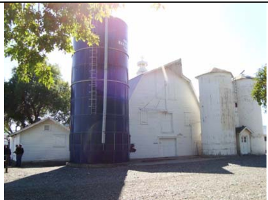
Bldg #3442 - Harvestore Silo
