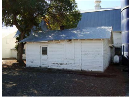
Bldg # 3467 – Drying Room East of Barn Complex
