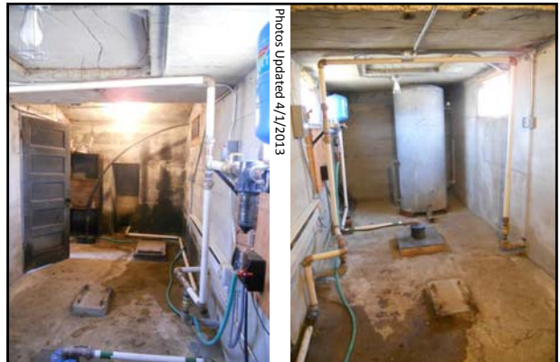
Bldg #3409 - Pump House
