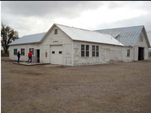
Bldg #3415 - Shop (attached to #3464 - Machine Shed #2)
