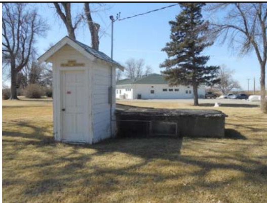
Bldg #3409 - Pump House
