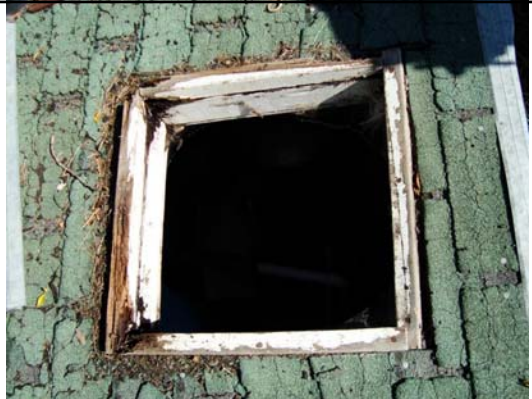
Pump House to Residences
