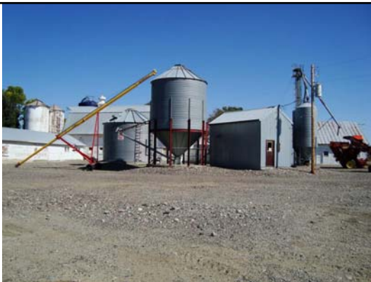
Grain Silos Southeast of Barn Complex
