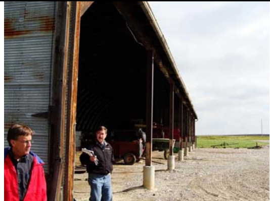
Bldg #3425 - Machine Shed #3
