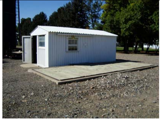
Bldg #3444 - Truck Scale House & Scale
