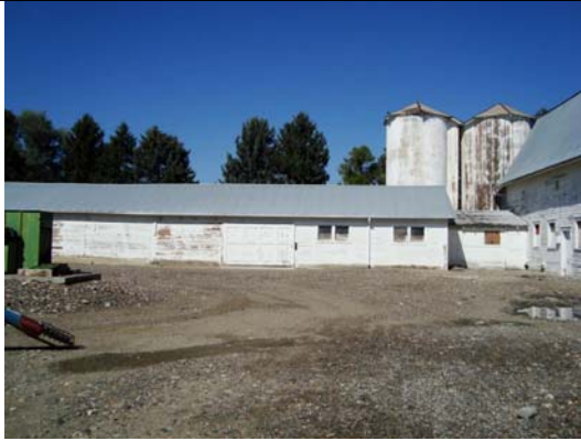
Bldg #3466 - Western Annex Barn Complex
