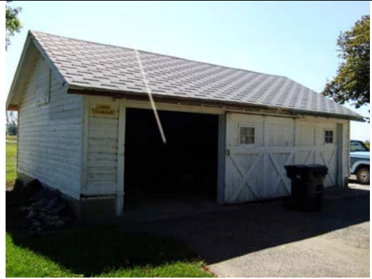
Bldg #3423 - East Residence Garage
