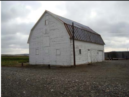
Bldg #3438 - Horse Barn / Machine Shed
