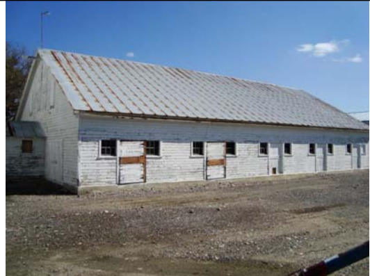
Bldg #3465 - Southern Annex Barn Complex
