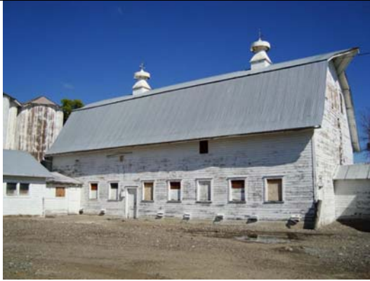
Bldg #3421 - Barn Center Condemned Section
