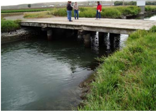
Bridge Over Canal (MSU owned)
