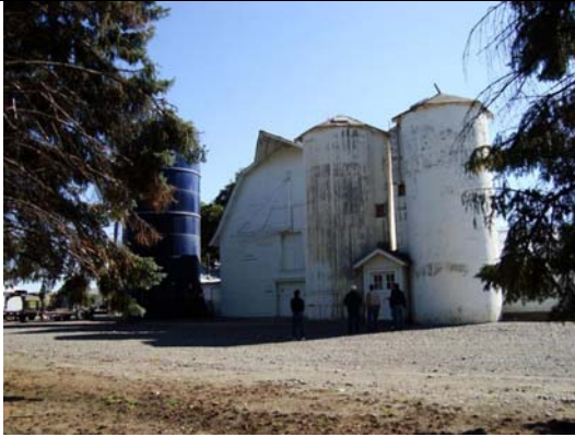
Barn Complex Entrance with 3 Silos of Different Materials -Bldg #3442 – Steel Harvestore Silo, and two Unused Silos (1 of concrete and 1 wood)
