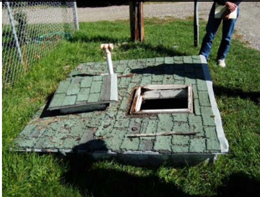
Pump House to Residences
