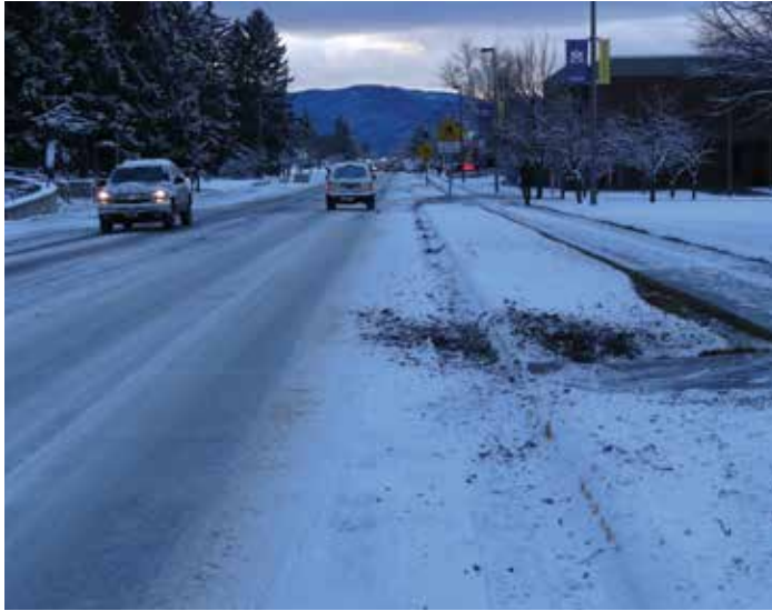
Bicycle Lanes are usually plowed after streets
