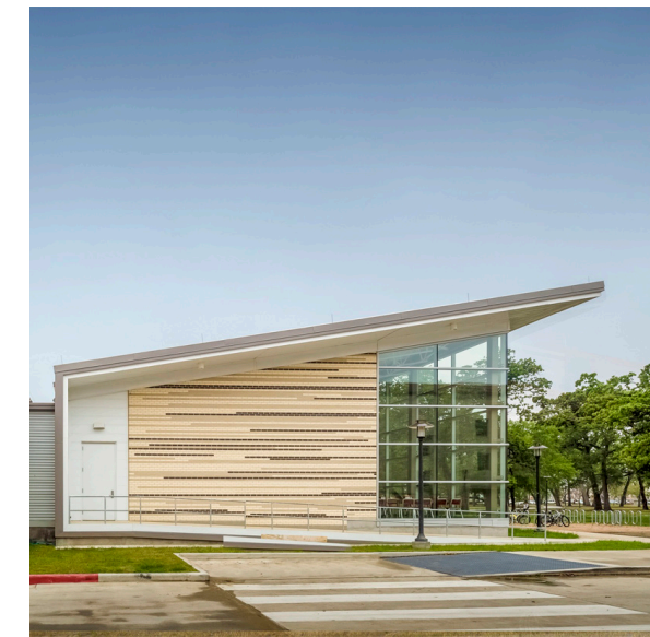
MASONRY AND GLASS
