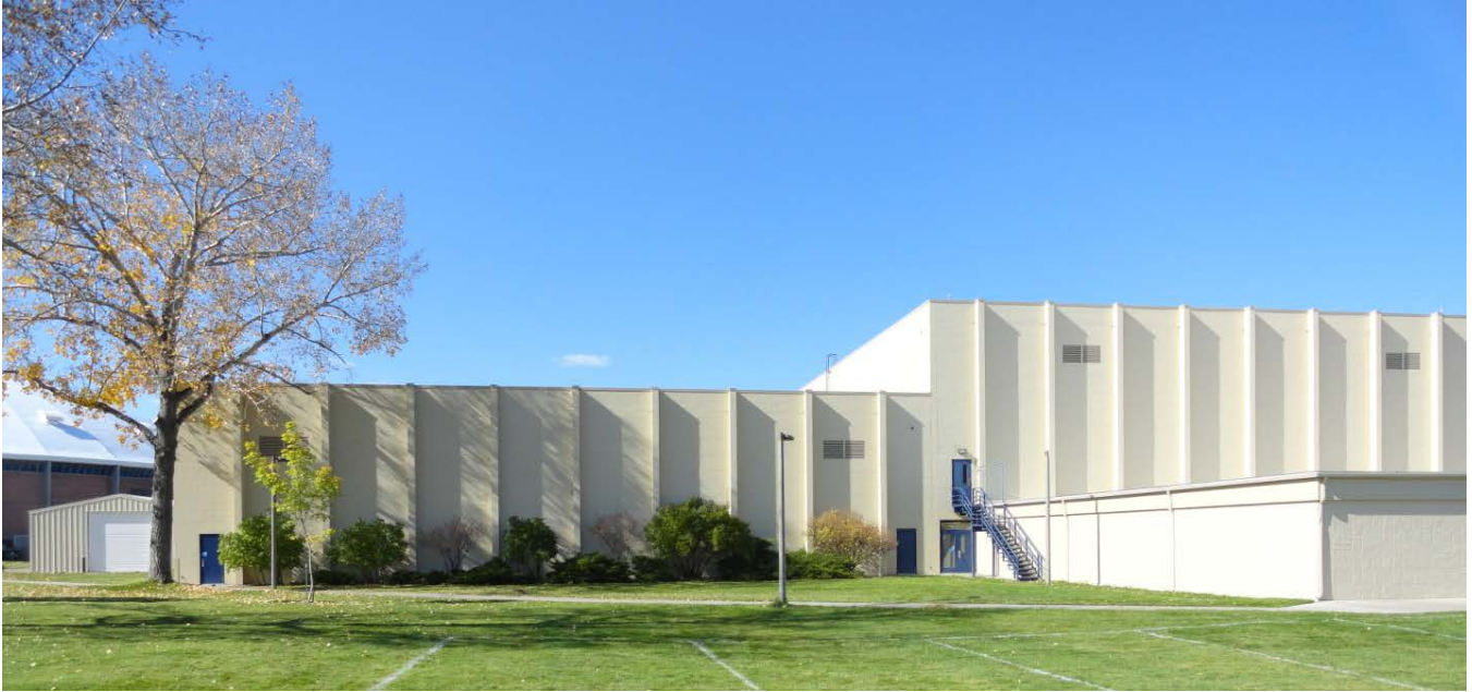
West view – Proposed EHHD Addition site at the Margo Hosaeus Fitness Center
