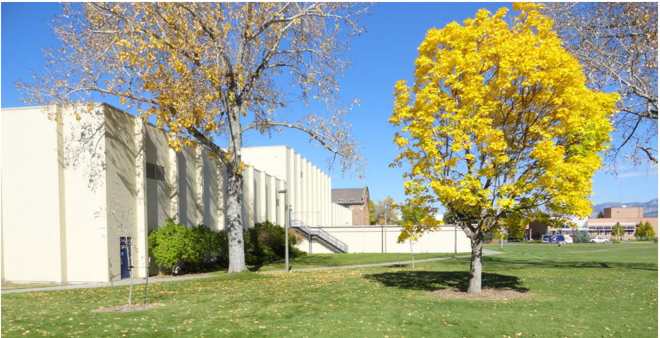
North View – Proposed EHHD Addition site at the Margo Hosaeus Fitness Center
