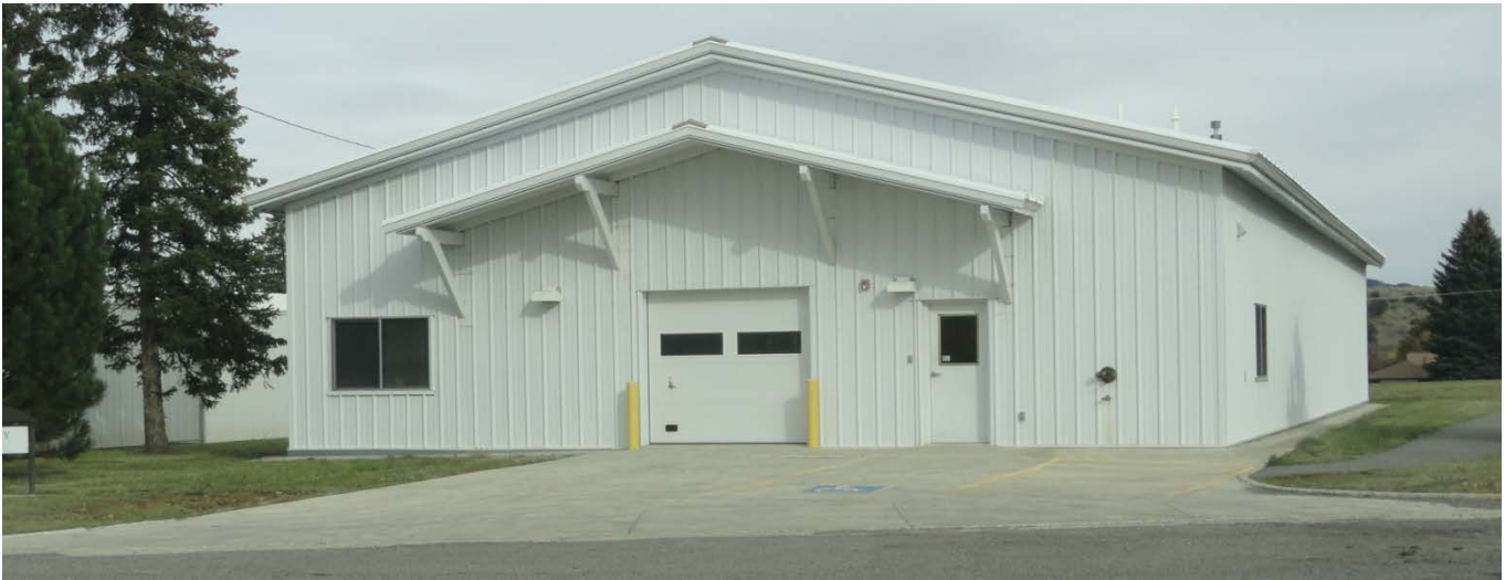
Records Management Facility (6,000 square feet, 50' x 120')
