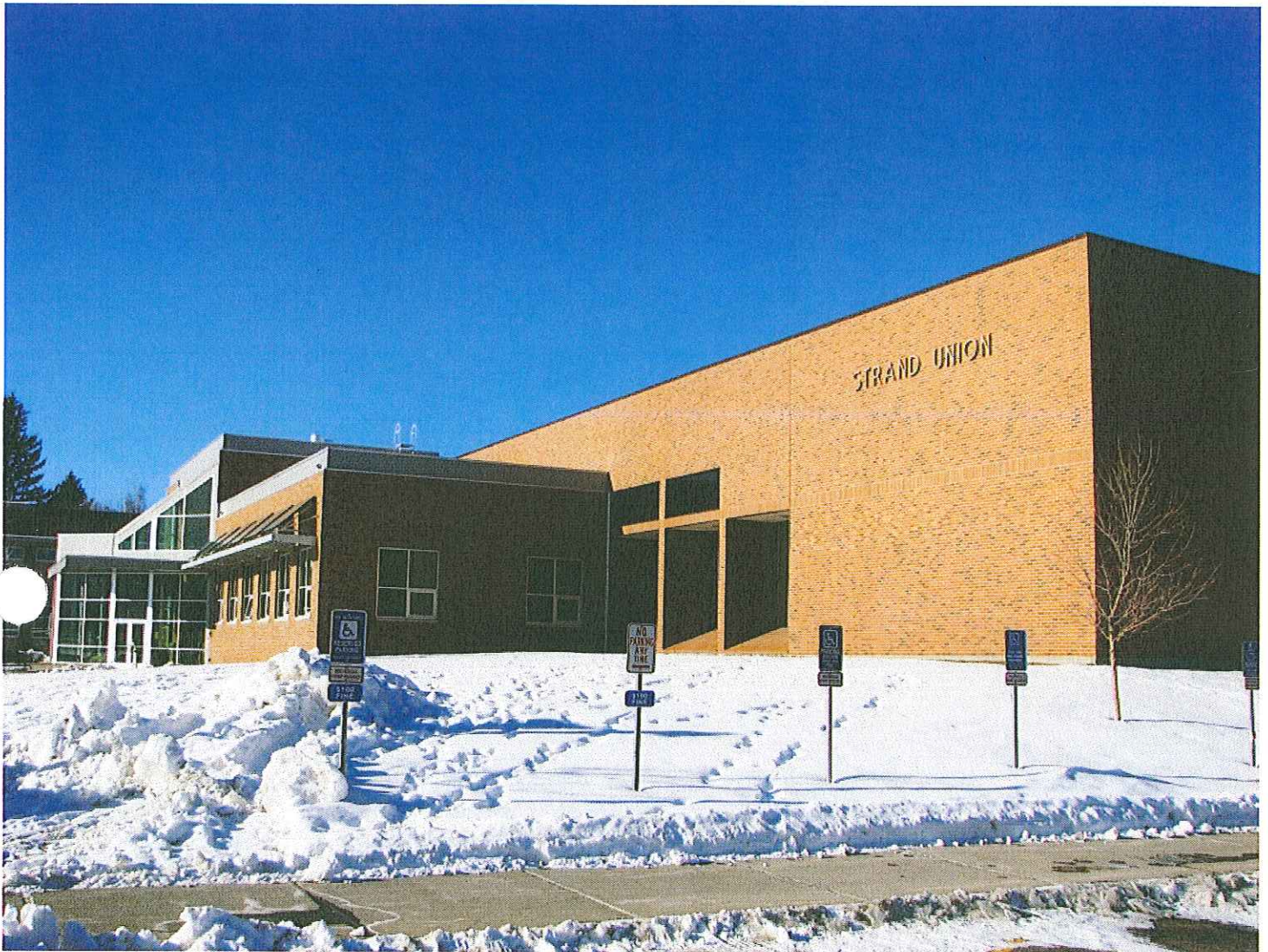
Student Union South Elevation with 2008 Addition (left) and 1983 Addition (right), Facing: NW Montana State University Jessie Nunn, January 5, 2013
