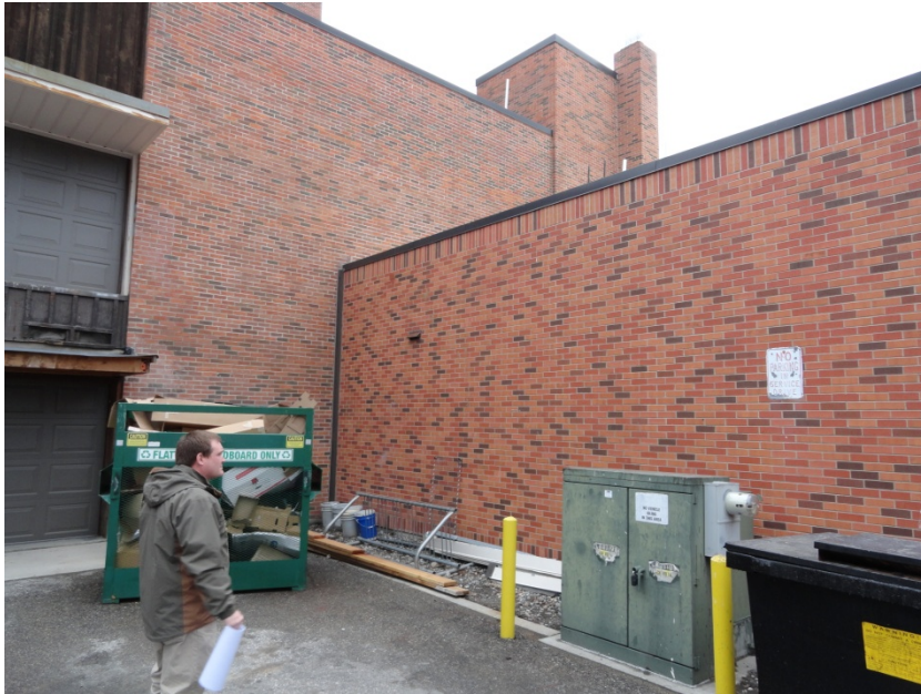
New door to the roof top of the Swingle Heath Center from 265ME
