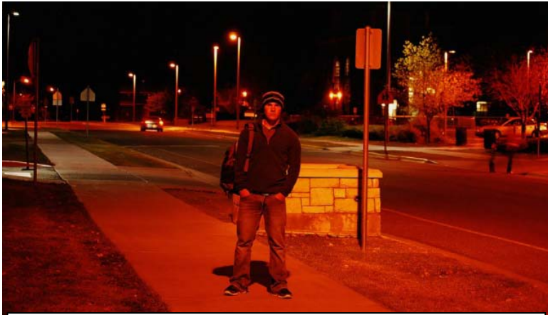
Under conventional high pressure sodium lighting, colors are hard to distinguish and light is delivered in a "blob" below the fixture, quickly diminishing with distance.
