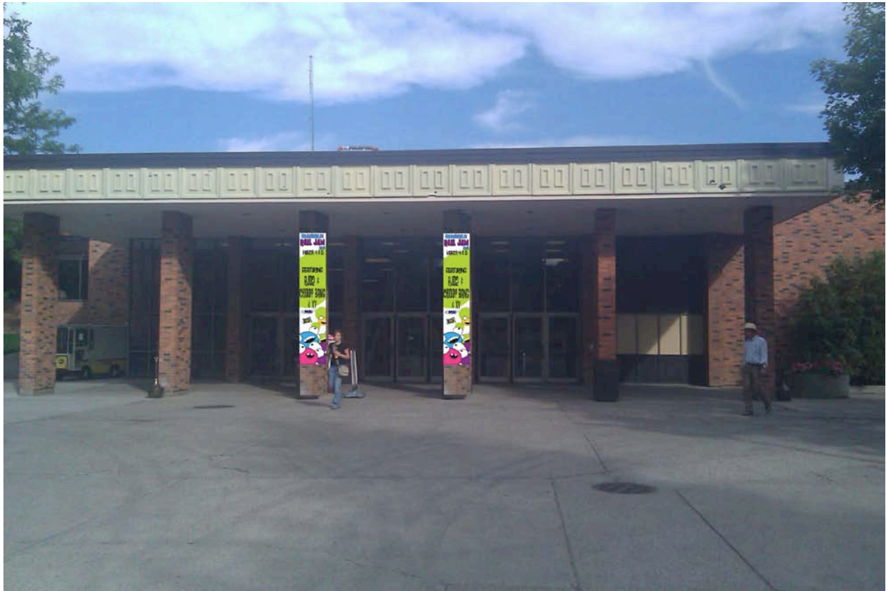
Example of proposed signage location on the west entry of the SUB
