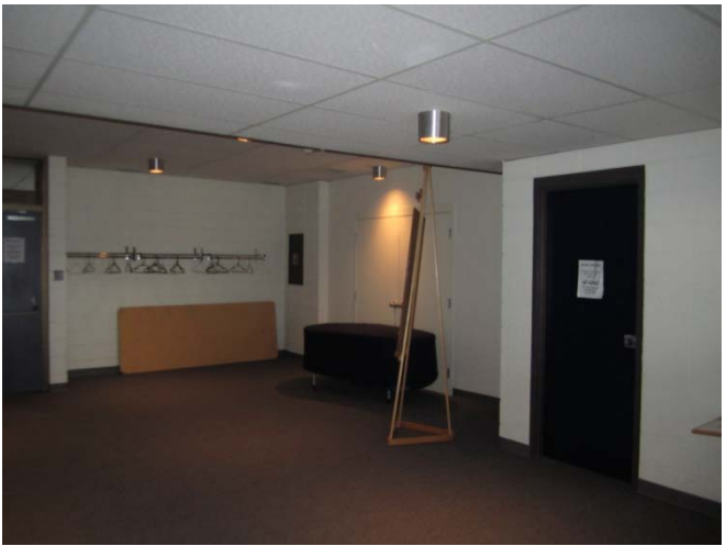
Existing storage area on north side of hall
